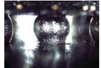
PBGA – cold joint: insufficient heat
