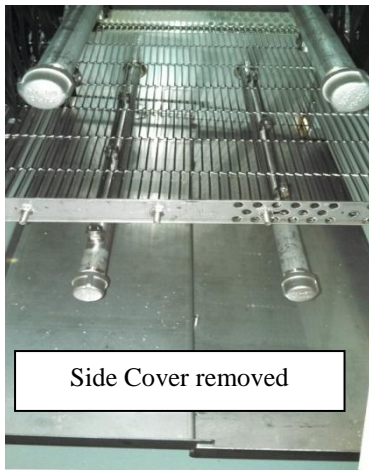
Figure 4: Pre-Wash Containment with Side Cover Removed
