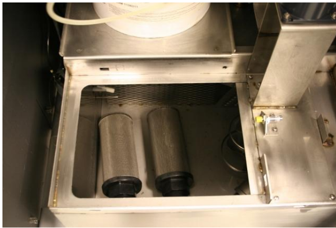
Figure 13: Batch Intake Strainers
