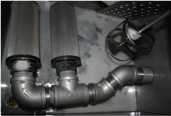
Figure 19: Batch Wash Tank after Draining out Wash Fluid
