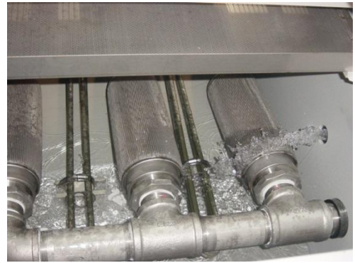
Figure 6: Strainers in Suction Inlet of the Wash Holding Tank
